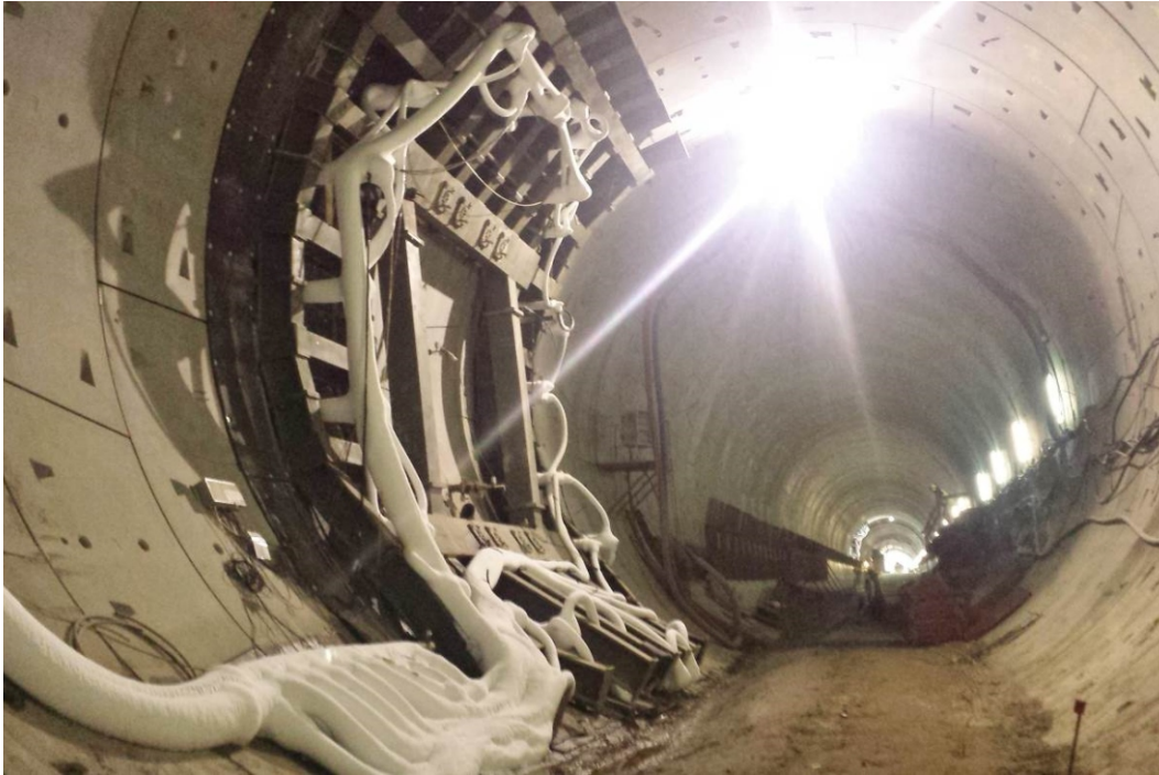
One cross passage in freezing stage
