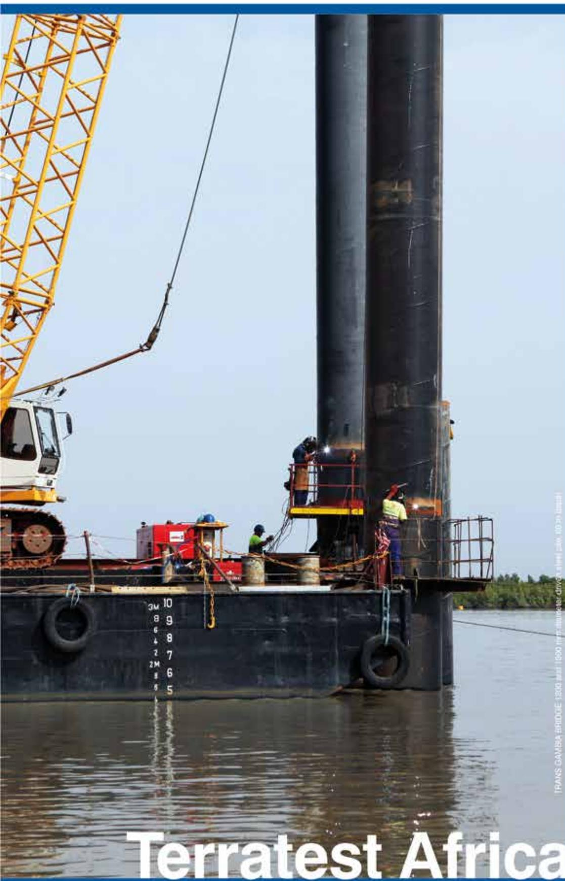
TRANS GARIBA BRIDGE | 1200 and 1600 mm diameter drive shafts | 40 m length
