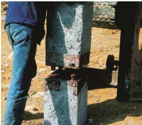
*Phase 1: Placing the pile for joining*
